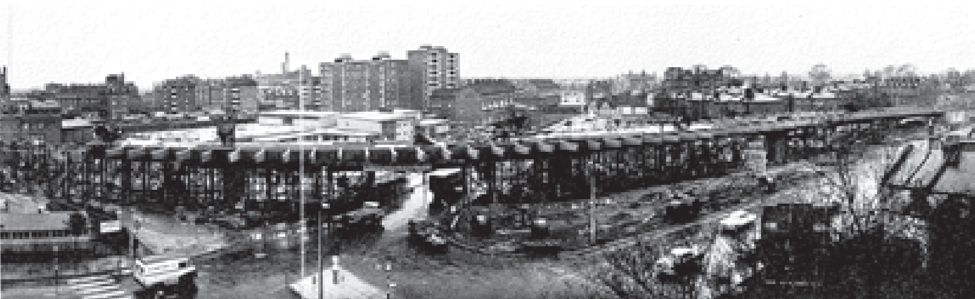
The last pre-stressed concrete segment was placed in position on June 21 1961, and the flyover was opened by the end of the year.
